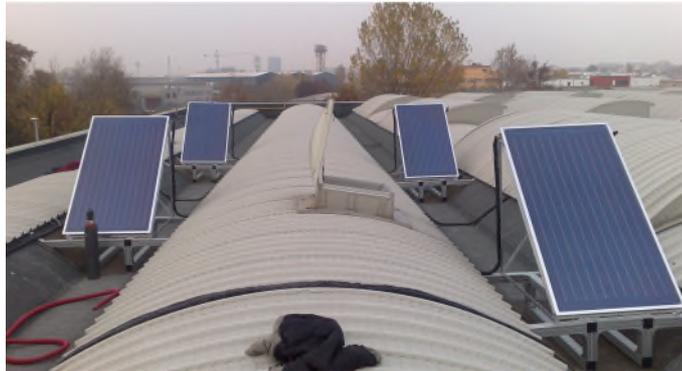
ESEMPI DI STRUTTURE REALIZZABILI CON ANGOLARI IN ALLUMINIO. SI POSSONO FORNIRE STRUTTURE CON DIMENSIONI 'CUSTOM'
